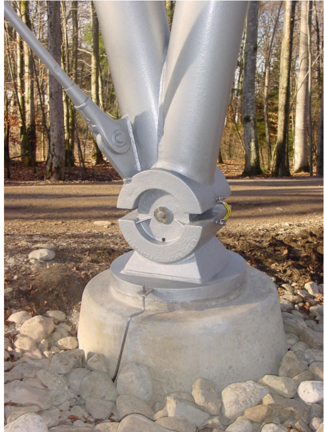
Cast steel knuckle-joints for the taking-over of thermal expansion.
