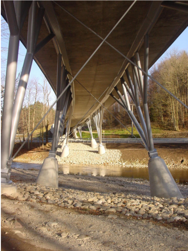
View from below the bridge
