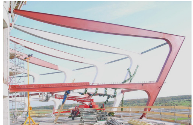
Beams spanning 17 m of unsupported length
