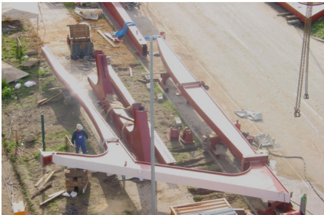
Pre-assembly with templates on site
