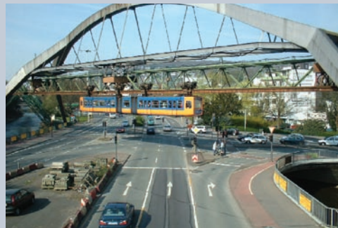
Suspended Monorail at Wuppertal/Germany: Test of MSM®-elements for 7 km sliding path/year at 30 mm/s
