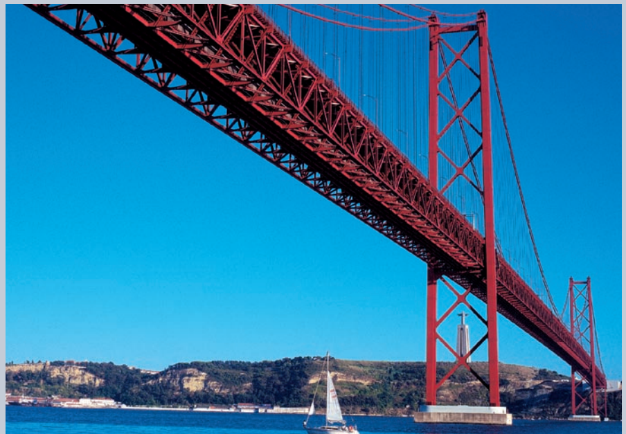
Tejo Bridge „25th April“, Lisbon/Portugal: MSM® Spherical Bearings for 10 km sliding path/year at 15 mm/s
